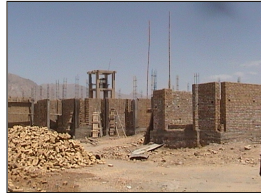
Construction work in progress
